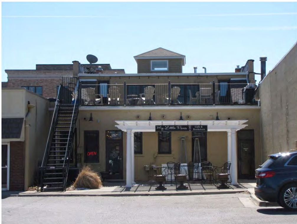
Main East 141-143_Looking South
