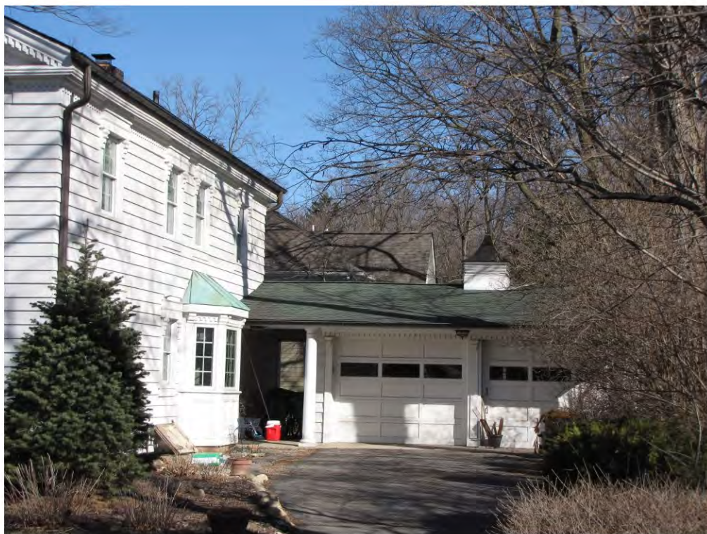
Randolph 204, Garage_Looking North
