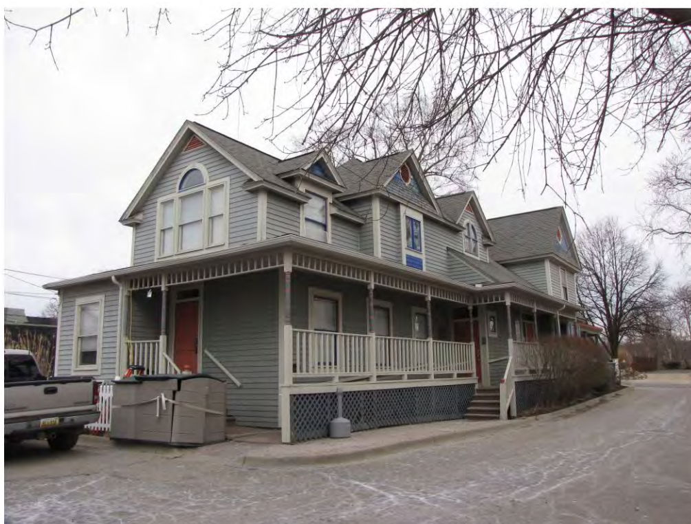
Main East 332_ Looking Northwest
