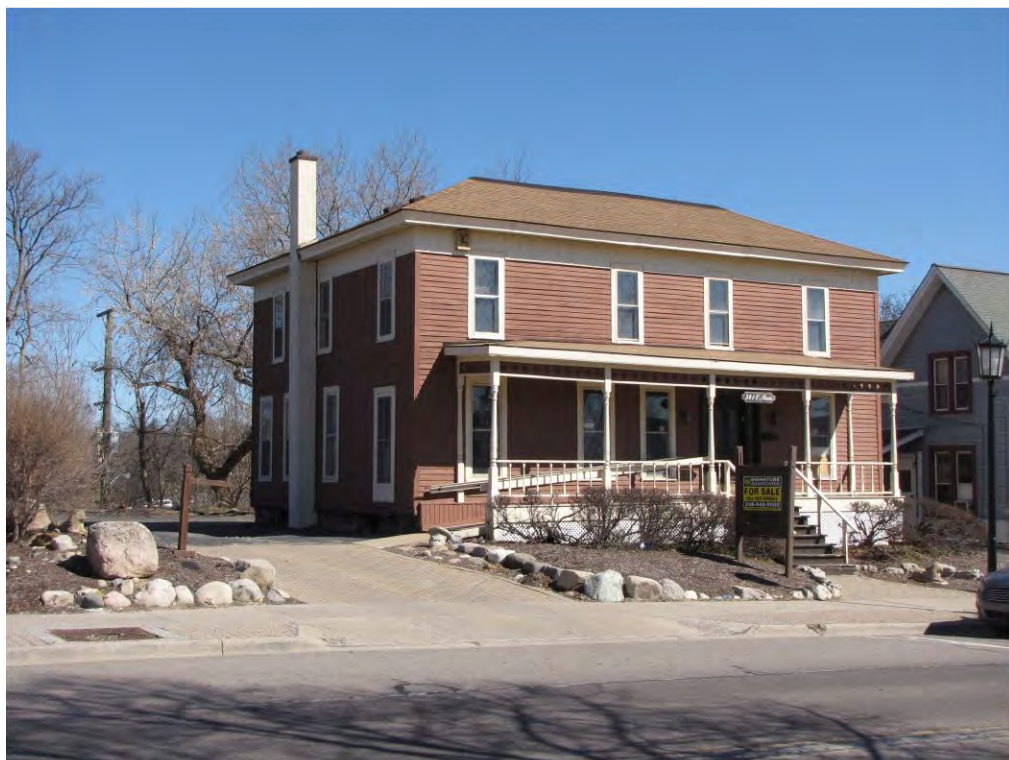
Main East 341_Looking Northeast
