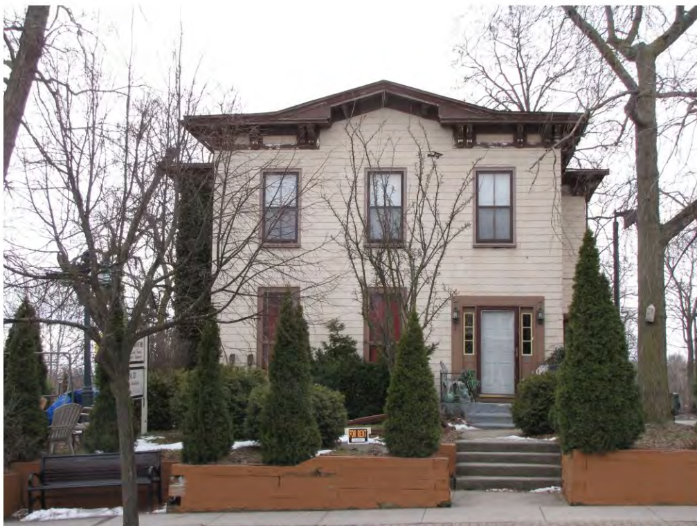
Main East 342_Looking South
