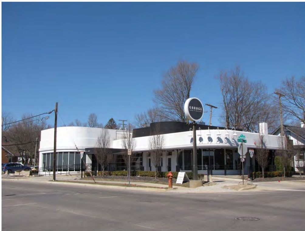
Main West 202_Looking Northwest
