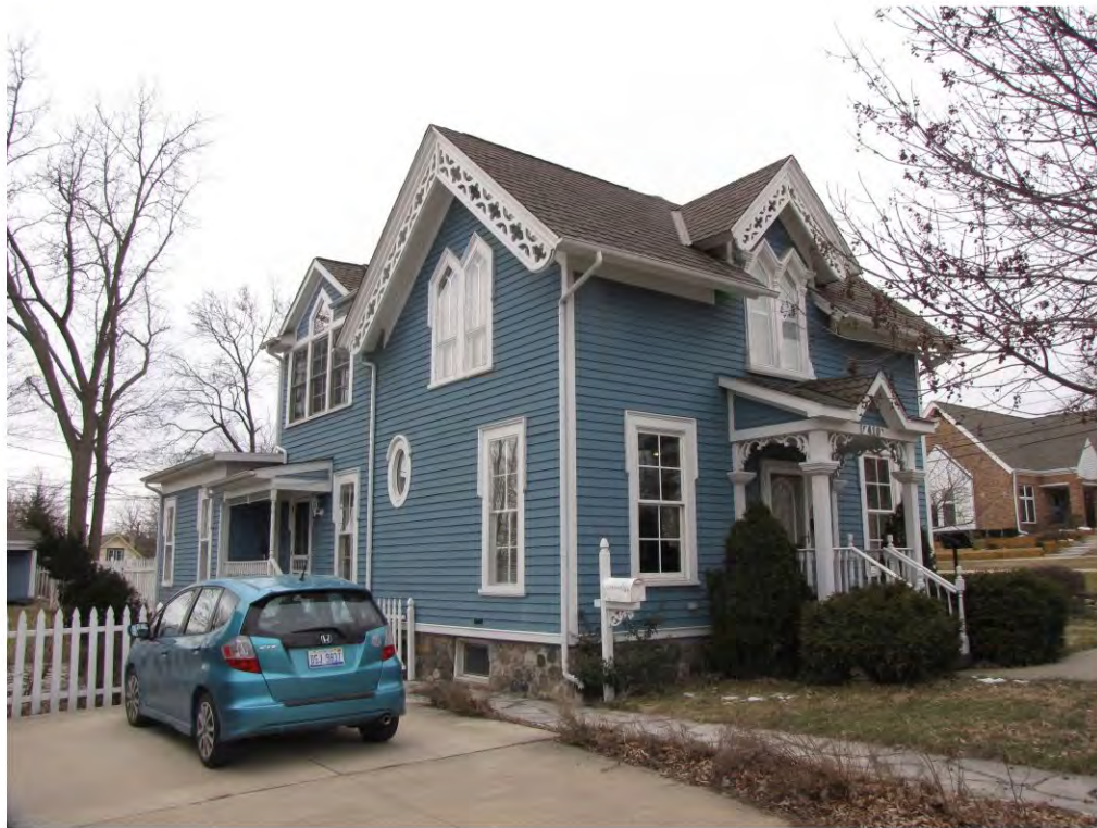
Main East 410_Looking Southwest
