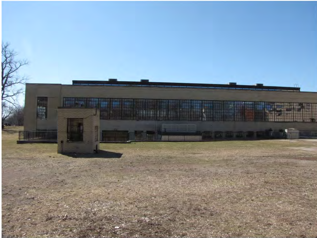
Main East 235_Looking South
