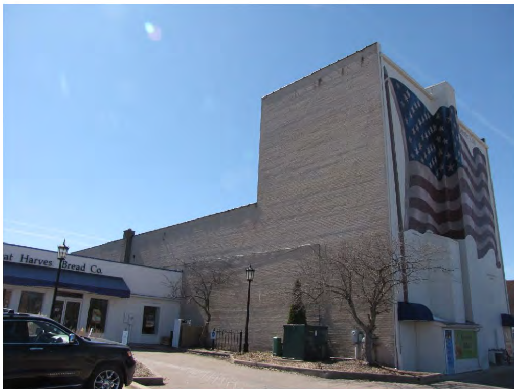
Main East 135-137_Looking Southwest
