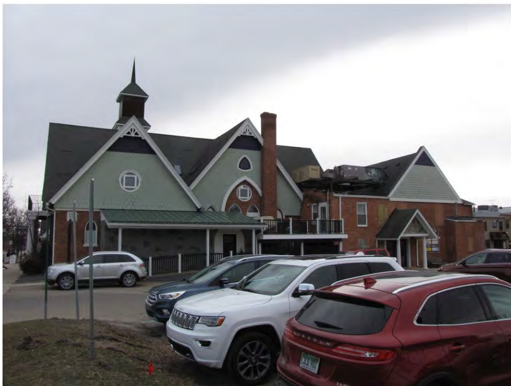
Center North 145-Looking East
