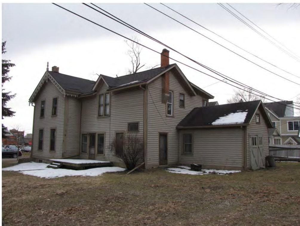
Wing North 129_Looking Southeast
