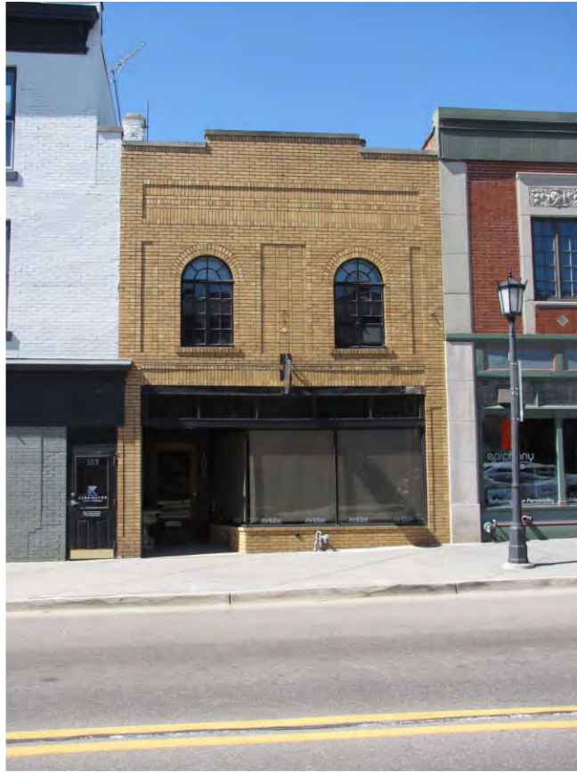
Center North 105_Looking West
