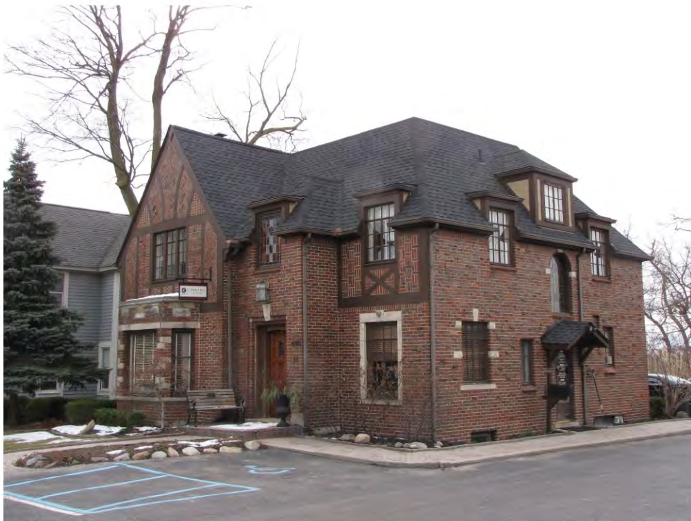
Main East 324_Looking Southeast
